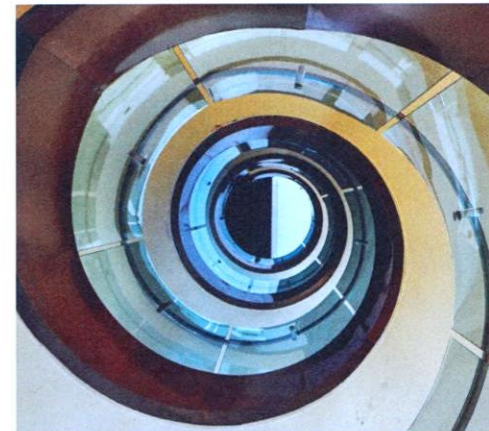
Sheets of tempered glass forms the tight inside curvature of the feature staircase's balustrade
