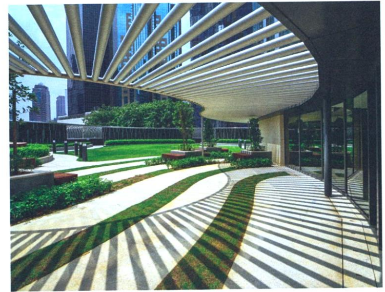
A curvilinear pergola of tubular members wraps over the podium façade, mirroring the landscape play in the hotel's outdoor function lawn
